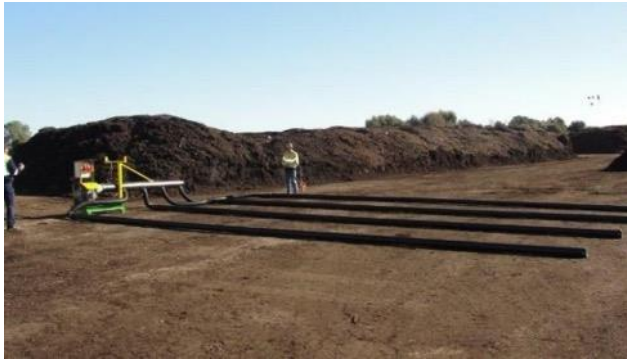
Photo 1: Aeration pipework laid out for a single module
